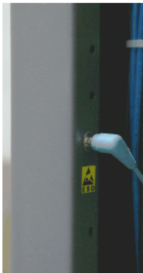
Figure 2-7 ESD jack on the N66E cabinet
