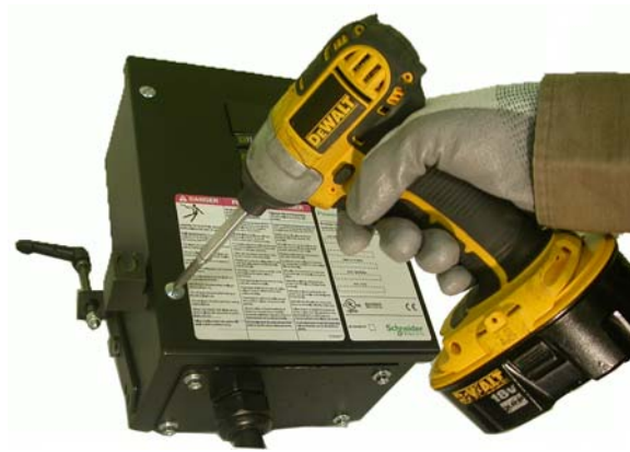
Figure 4: Securing the Plug-in Unit Cover, Back and Bottom (PBPQOD, PBPQHD)
