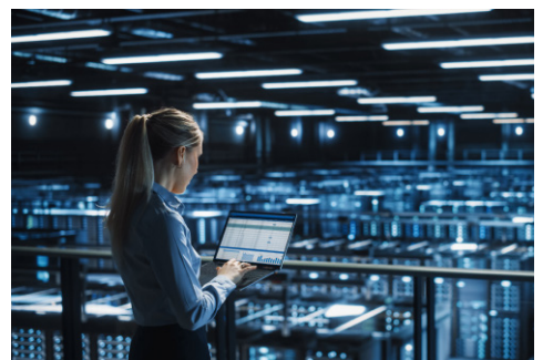
Micro Data Center & Server Room
