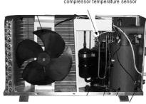
Figure 27: Compressor temperature sensor.
