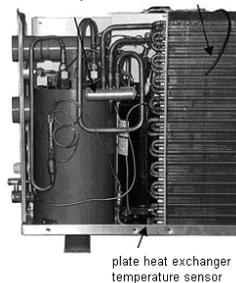
Figure 26: Plate heat exchanger temperature sensor.
