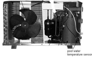
Figure 24: Pool water temperature sensor.
