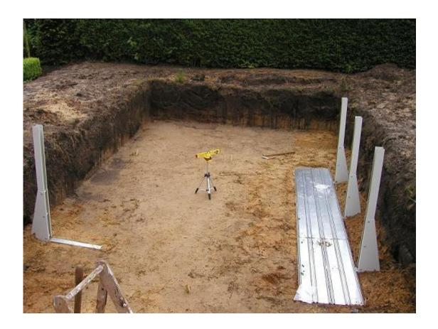
When all side supports are adjusted according the instruction, it is time to equalize/fill up the floor with sand and Styrodur isolation plates and/or make the final concrete floor.
