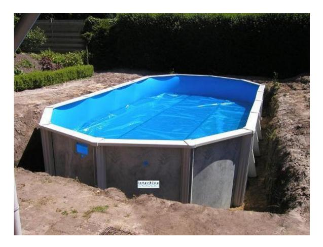
On this picture mounting the liner has been finished. But you can only start finishing the liner when there is about 60–70 cm of water in the pool. Not sooner, because the liner may shift a little during the filling process.
