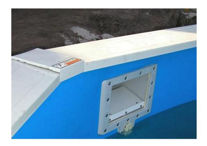
The pool is nearly finished. Fill the water just under (5–10 cm) the inlet and skimmer edge.
