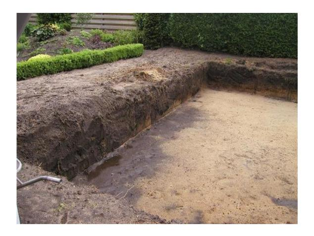
It all starts with the digging of a hole with a nice (water) leveled floor below. Always excavate the hole a bit larger than the size of your pool. We recommend about 50 cm larger on all sides (for a pool sized 8.50 x 4.90 m a hole of at least 9.25 x 5.75 m should be excavated)
