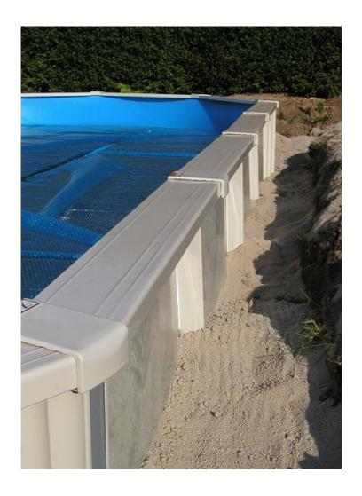
When skimmer and return fitting are mounted, fill your pool till 5 cm below the top edge. After this you can start re-filling the hole in which the pool is built. (Also look at step 3, excavation drawing.)
