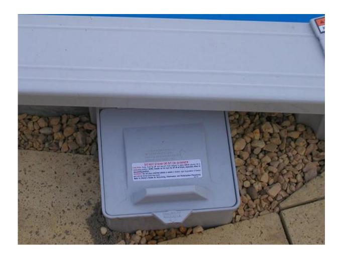
Because you built the pool a little above ground surface level, the skimmer lid fits perfectly in the pavement.
