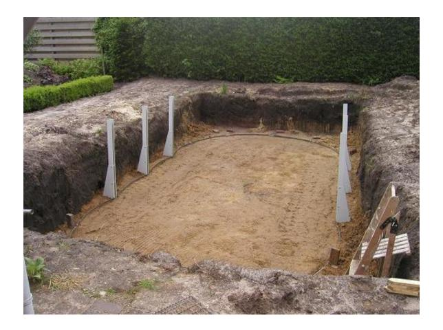
The picture below shows a floor of sand. This could also have been a concrete or a stabilized sand floor.
