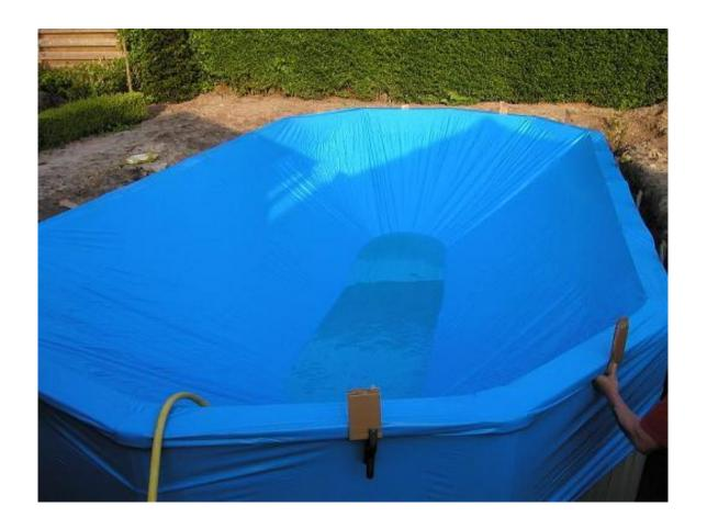
The casing of the pool liner can now begin. Carefully read the instructions on how to do this. We see here that the liner is first hung over the pool all around until the bottom seam is around 30 cm under the edge.
