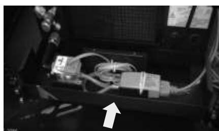
Figure 3-18 Installation of the pump kit
