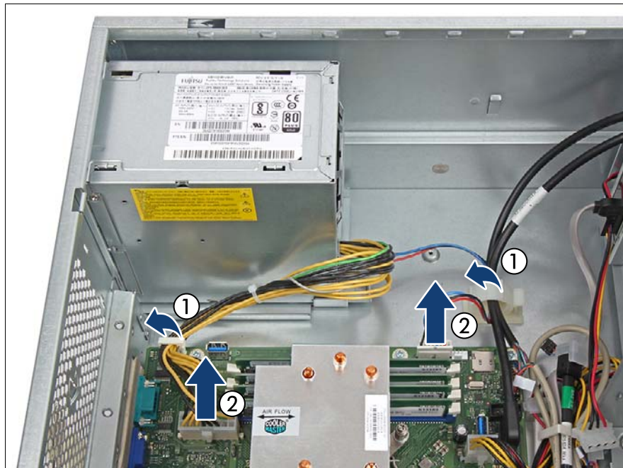
Figure 56: Disconnecting the power cables
