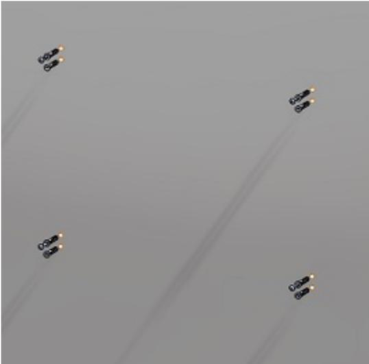
7. Screw one M5 screw on each corner, four screws total, into the anchors, leaving approximately 5 mm (0.20 in) gap between the anchor and the screw.
