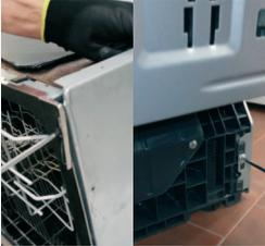
2. By using the 15 pipe wrench, remove the screws that fix cabinet cover
