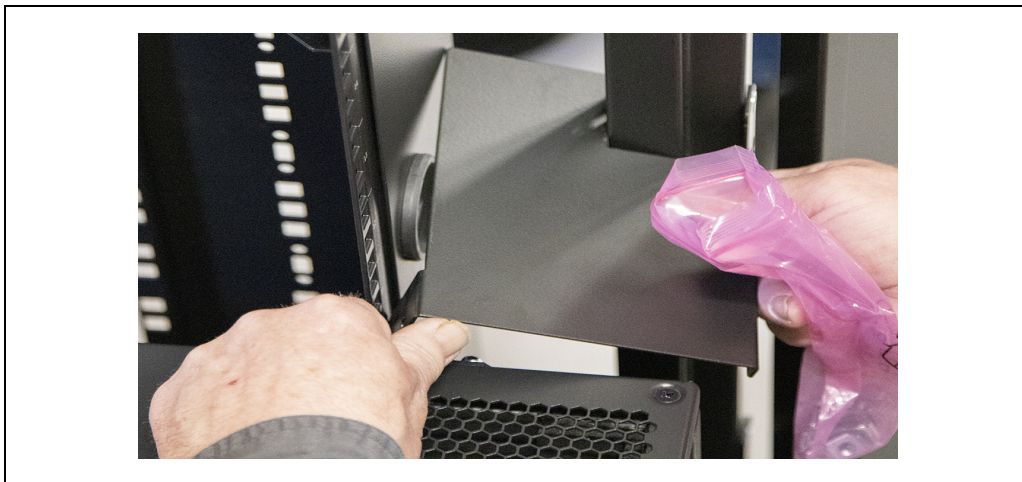
Figure 4.2 Attach Air Baffles—800 mm (31.5 in.) Rack
